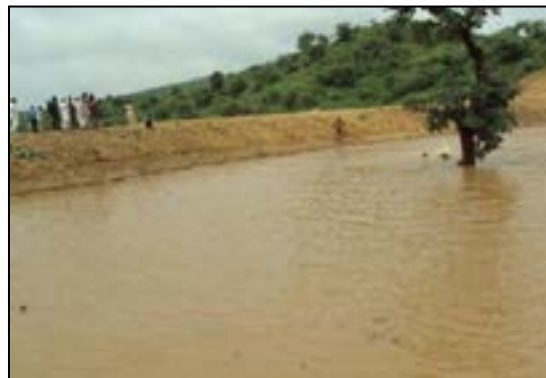
Earthen Check Dam (Paal)
